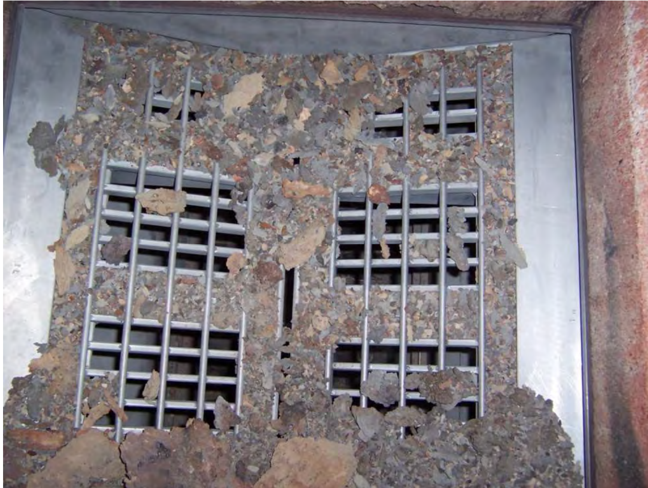
Grid Doors Installed at SCE&G McMeehin Station
