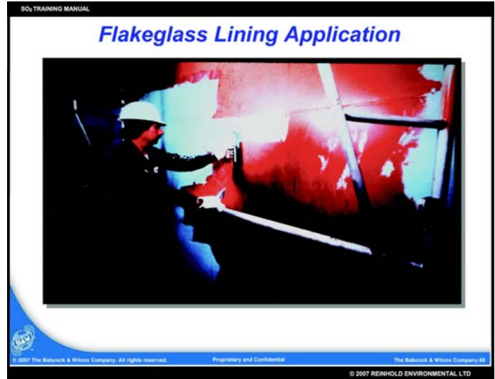
Flakeglass Lining Application
