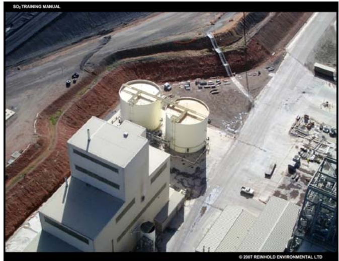
Bulk Slurry Storage Tanks Used with permission
