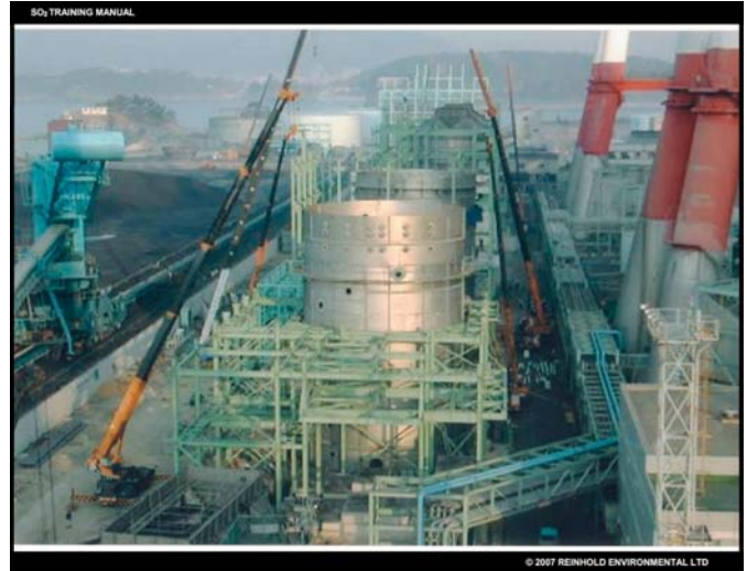
Absorber Erection Used with permission from Korea Cottrell Co., Ltd.
