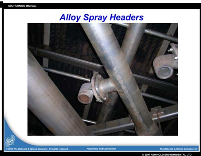
Spray Headers - Alloy Used with permission from Babcock and Wilcox
