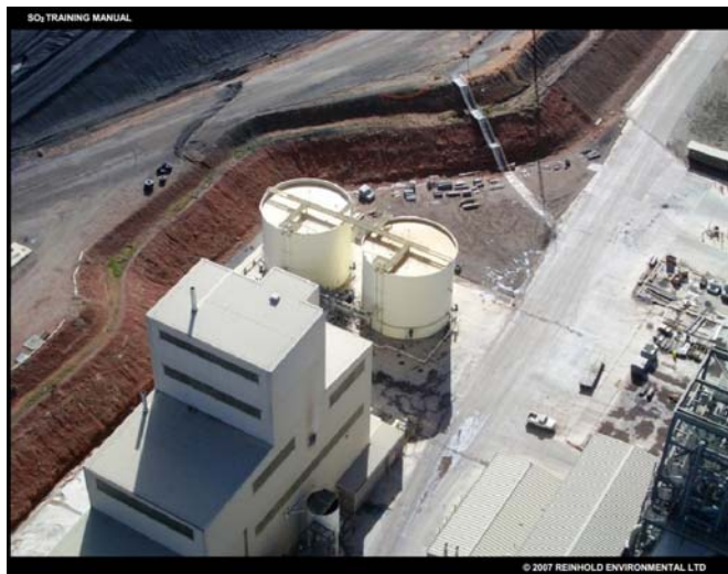
Bulk Slurry Storage Tanks Used with permission
