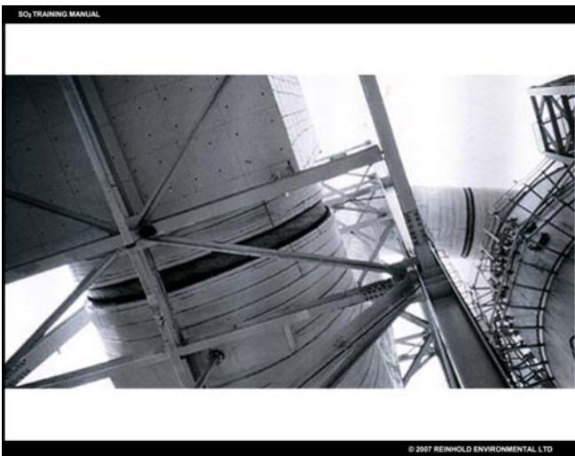
Expansion Joint Installed in Duct Used with permission
