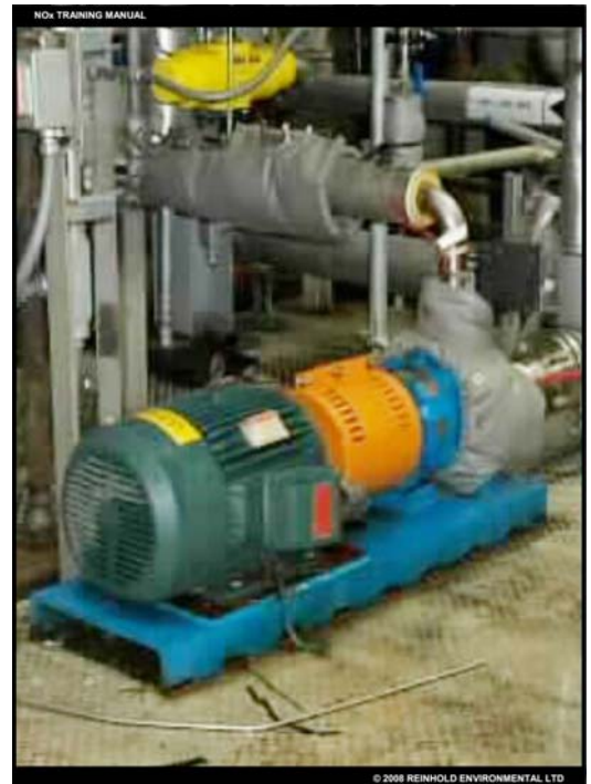
Urea Solution Pump (Used with permission)
