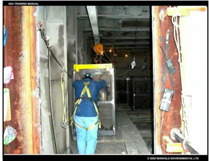
Catalyst Module Entering Reactor (Used with permission)
