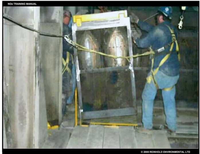
Loading Catalyst Transfer Cart (Used with permission)
