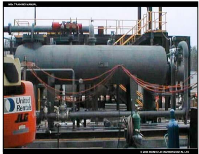
Aqueous Ammonia Vaporizer
