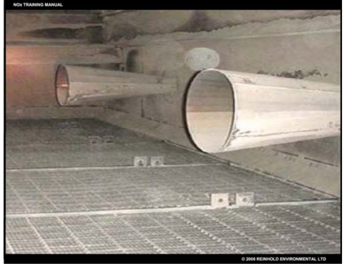
SCR Airhorns (Used with permission)
