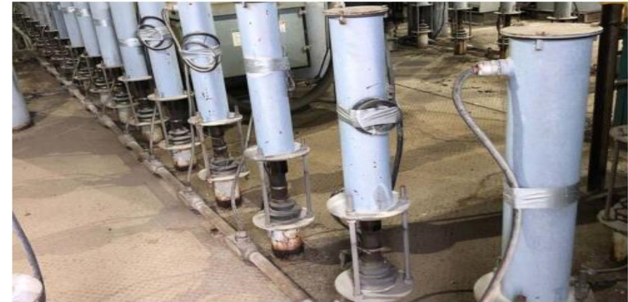
Collector Plate Tumble Hammer Rappers
