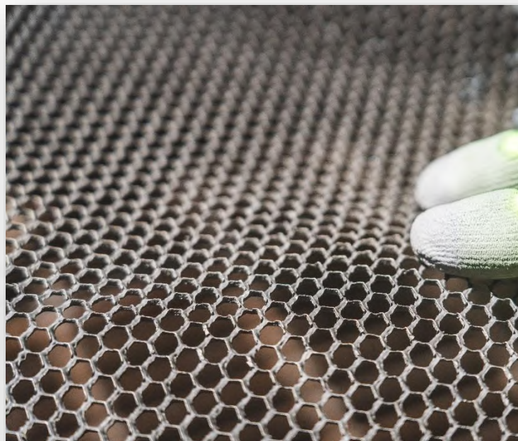
Screen End of Life – Replace ASAP
