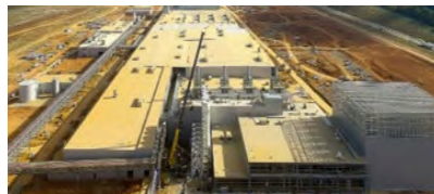
Hankook Tires Concrete designed with CUF Fly Ash
