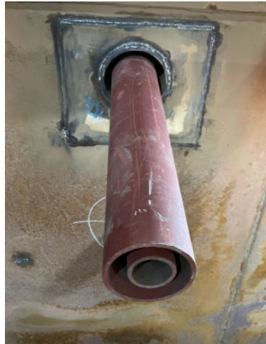
Five (5) Large Bore Pipe in a Pipe Injection Lances
